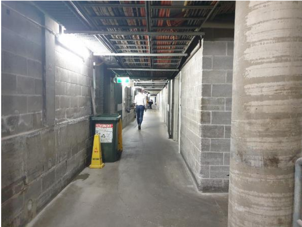
Figure 15: Common building service corridor
