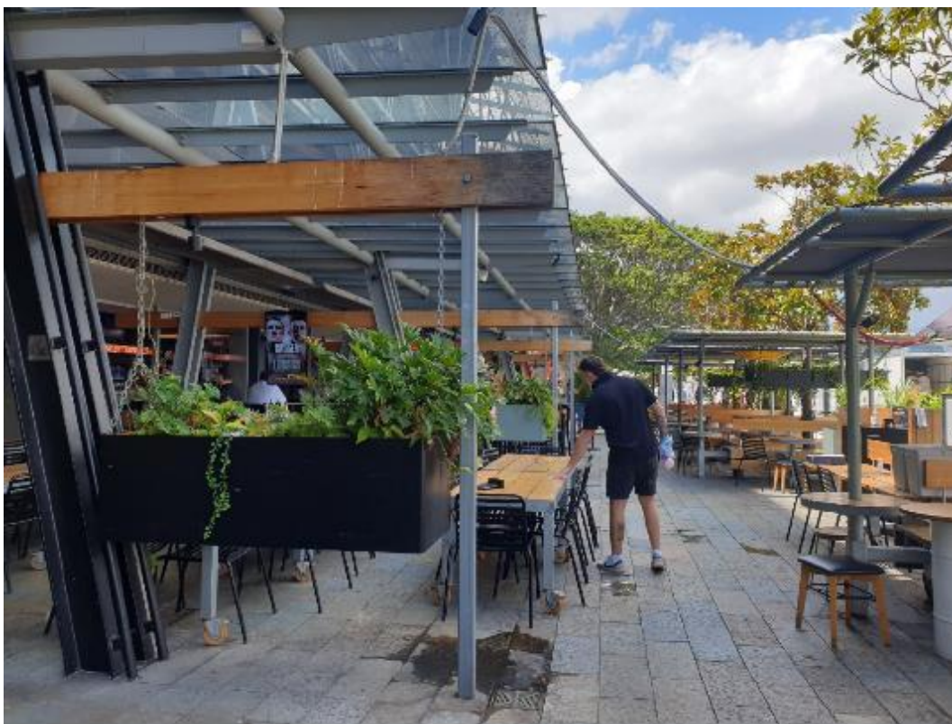
Figure 5: Looking south at outdoor seating area of subject tenancy
